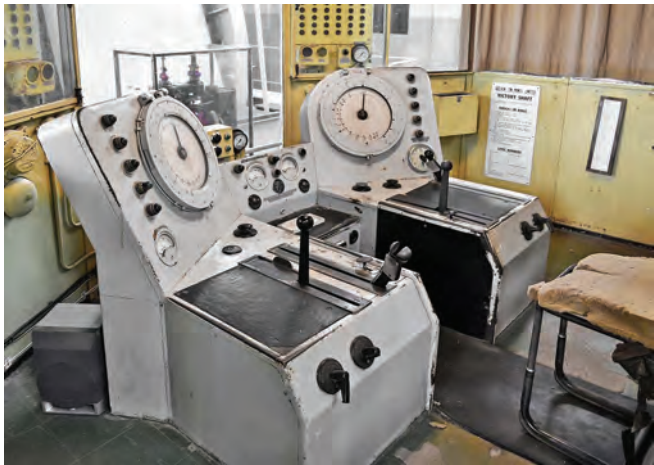
Victory Shaft cage controls. Photo Ken Geddes
